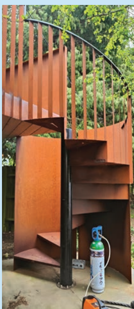
Spiral staircase in Cor-Ten steel
