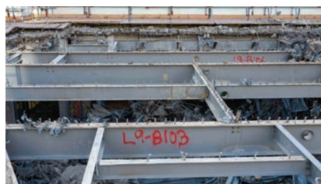
Figure 3: Steelwork during demolition and recovery (Courtesy: Elliott Wood)
